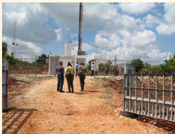
Site visit being conducted at the remote monitoring site at Planters Hall, St. Catherine.
