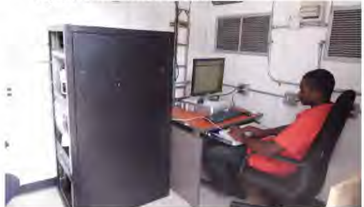
Telecommunications Engineer, Philmore Trowers at the new remote site.
